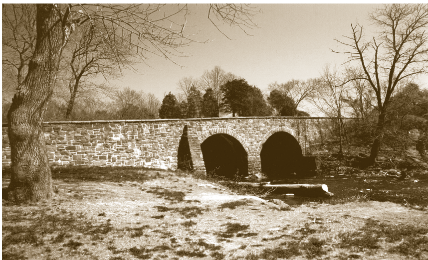
▲ Bridge at Bull Run
