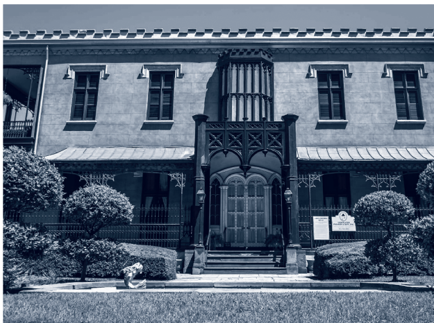
◀ The Green-Meldrim Home in Savannah, Georgia
